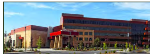
Fort Hall Casino Expansion
