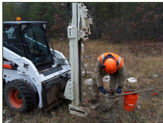
Sampling activities at the former Old Gun Range/Illegal Dump site
