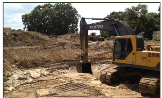
Excavation and stockpiling activities at the Red Barn property
