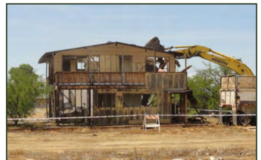
Properly demolishing buildings with asbestos containing material at the old feed lot brownfield site
