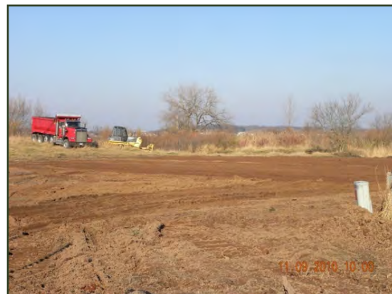
Excavation activities at the Eastlake property
