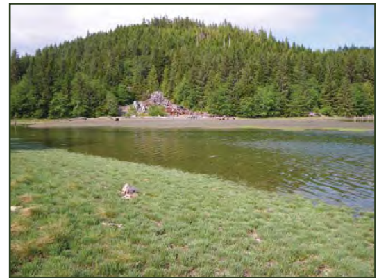
Dilapidated structures at the Salt Chuck Mine site as seen from across Ellen Creek
