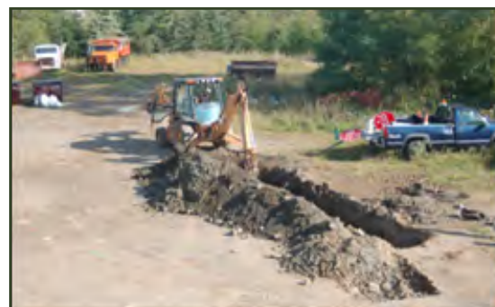
Phase II test pitting activities conducted at the Passamaquoddy Public Works Garage Site
